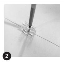
Fix clips with suitable screws.
